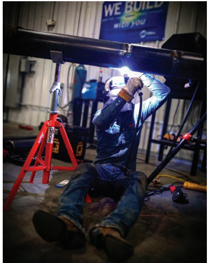
Fig. 2 — An instructor demonstrates a gas tungsten arc welding cover pass in the school's pipe lab. AWA believes confidence is built both in the booth and while welding in typical field settings.
