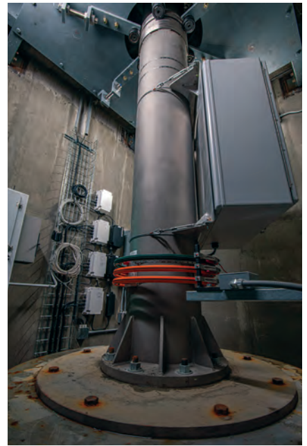
Fig. 2 — Custom Koike turntable fabricated to support and continuously rotate the 40-ft statue of Genesis.
