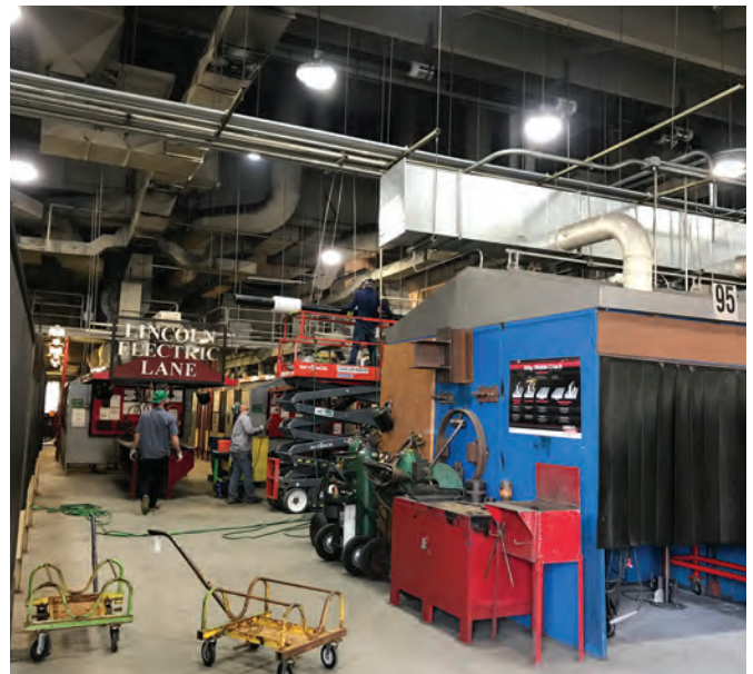
Fig. 4 — Pictured is PCC's Rock Creek Campus welding shop prior to renovation, which is currently underway. When the college's students return to in-person learning in spring 2021, they will be welcomed with a new state-of-the-art facility.
