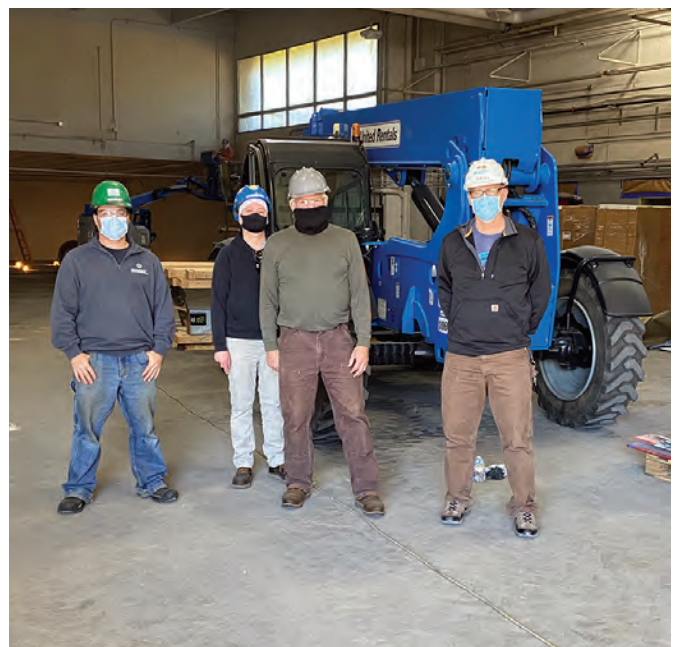
Fig. 5 — PCC Welding Instructors (from left) Dave Williams, Lauren Cobb, Scott Judy, and Matt Scott gear up in PPE to help with the school's welding shop renovation.
